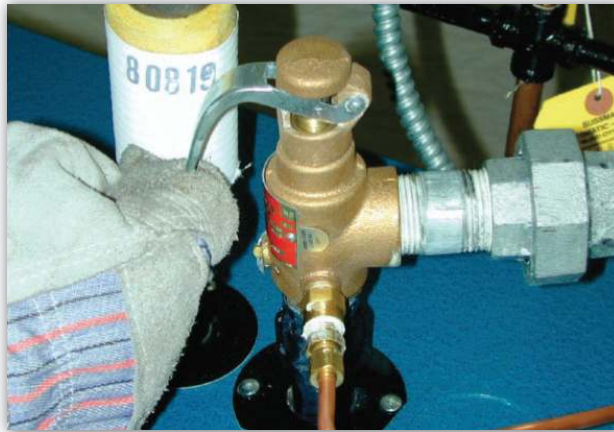
Testing a Steam Release Valve
